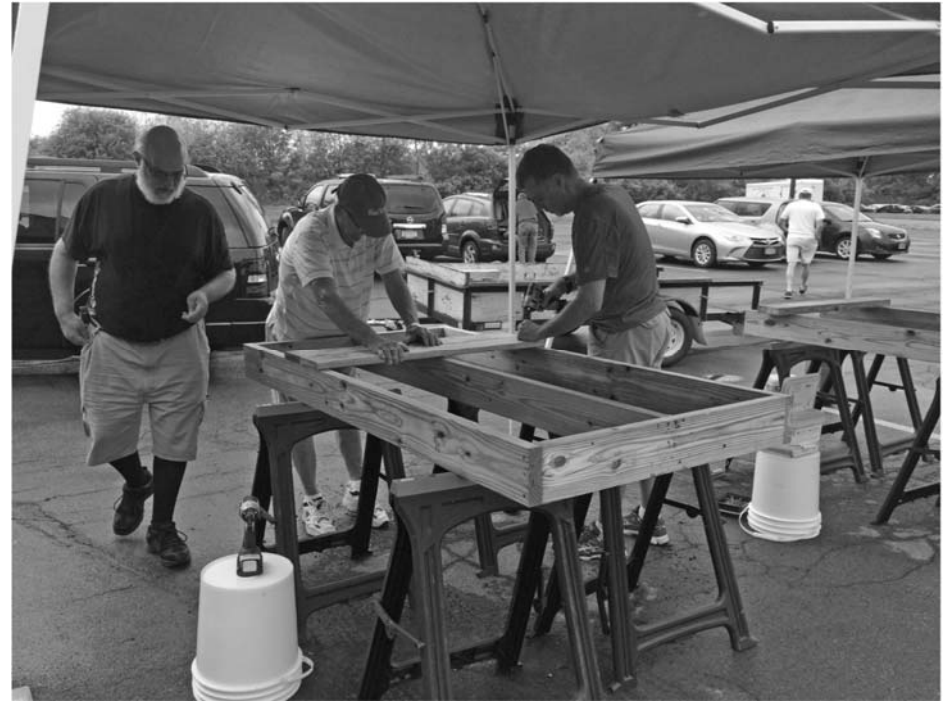
Pictured is Upper New York Area Resident Bishop Mark J. Webb helping Operation Northern Comfort volunteers build ramps.
